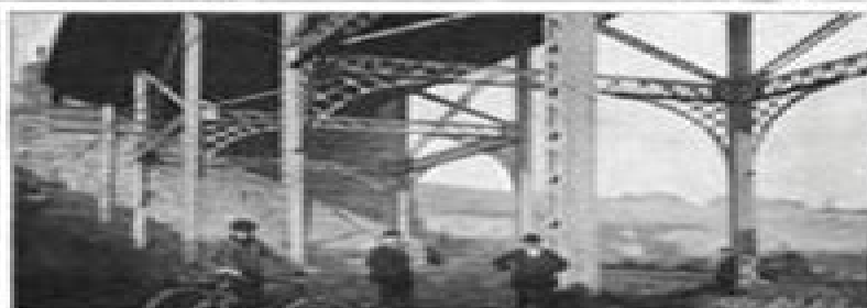
REMARKS THE LONG SPAN OF THE BRIDGE, SHOWING WALL OF THE BRIDGE AND BRIDGE AND BRIDGE.
