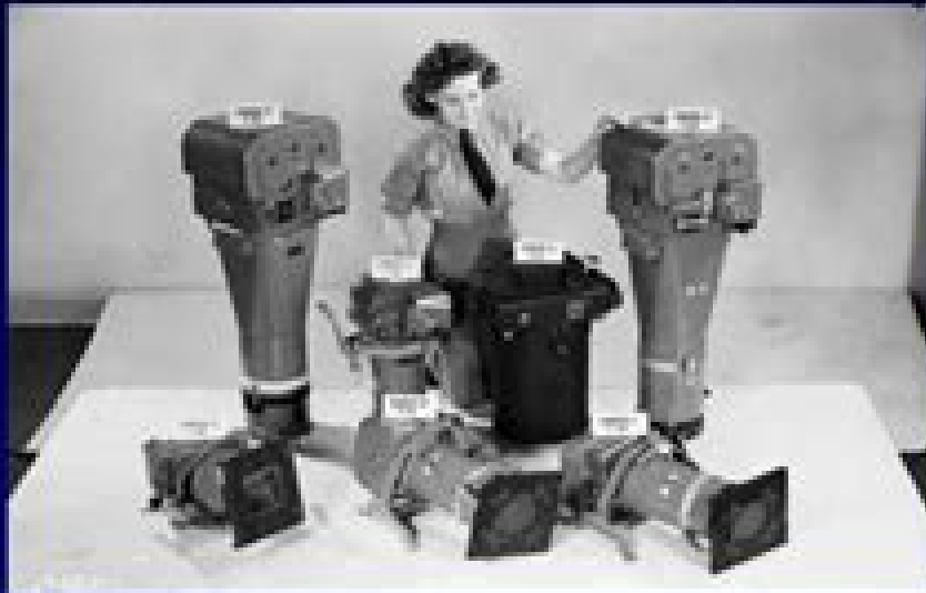
Types of aerial photographic cameras used by the RCAF in 1945 Public Archives Canada Photo PA- 065562
