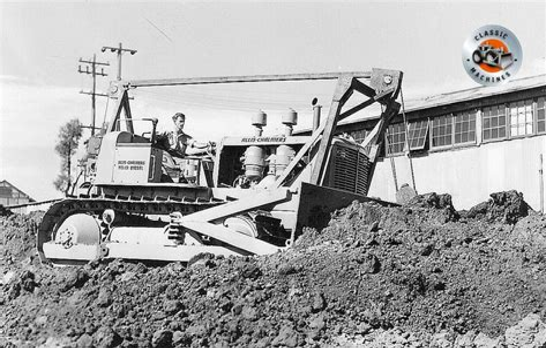
This Allis-Chalmers HD-19 is fitted with a LeTourneau AK8 angledozer and rear mounted LeTourneau PCU.
