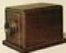
1880 First Commercial Telephone: The first, commercial telephone, shown at the 1880-1881 World's Fair in London.
